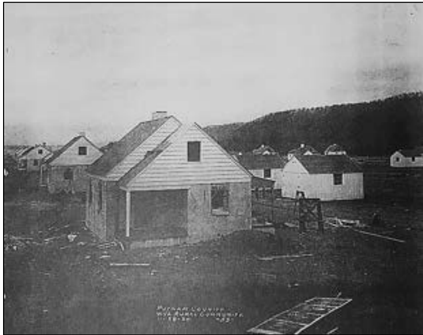
Figure 8. Dwellings and Barns during Construction, 28 November 1934. Source: FERA.
