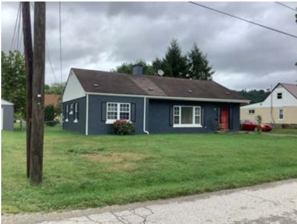
Photograph 26. PU-0007-0105 at 210 Chestnut Street, facing Northeast.
