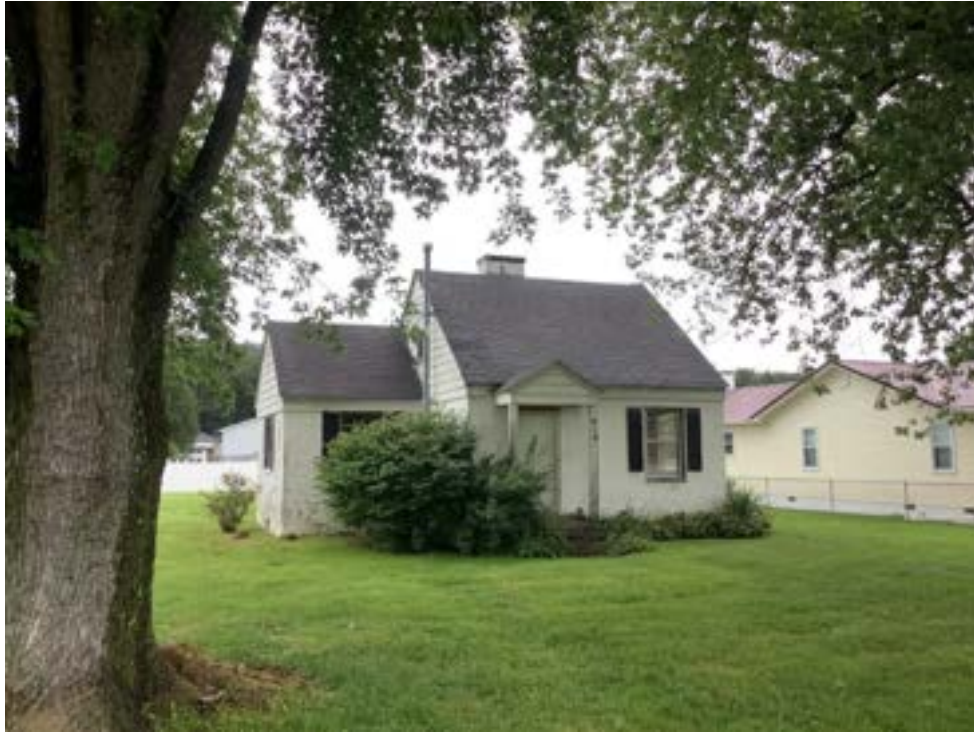
Photograph 23. PU-0003-0417 at 942 Roosevelt Boulevard, facing North.
