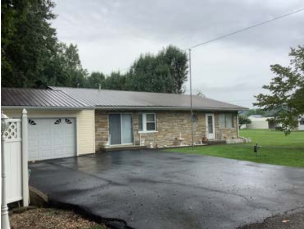
Photograph 27. PU-0007-0170 at 122 Kapok Street, facing South.
