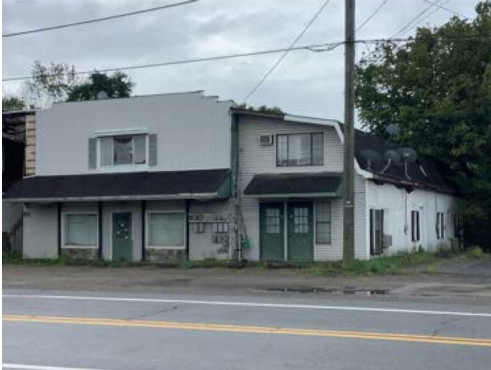
Photograph 17. PU-0007-0149 at 935 Roosevelt Boulevard, facing South.
