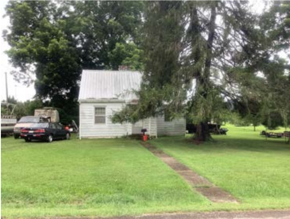
Photograph 19. PU-0003-0365 at 302 Ivywood Street, facing Southeast.
