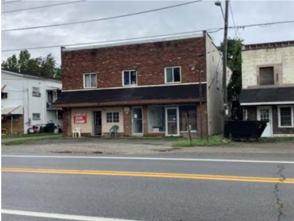
Photograph 15. PU-0007-0148 at 833 Roosevelt Boulevard, facing South.
