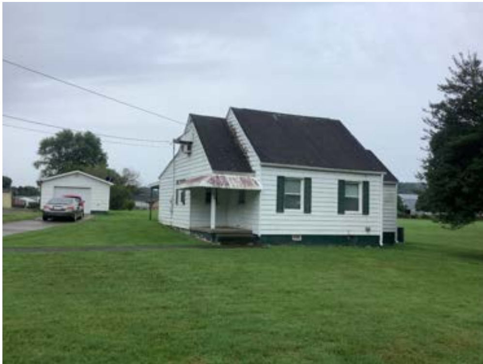
Photograph 22. PU-0003-0399 at 116 Kapok Street, facing South.
